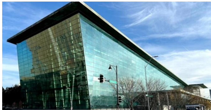
Figure 2: Patmos AI Campus (former printing press building).
