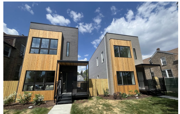
Modular homes constructed in Chicago (Photo: Block Club of Chicago)
